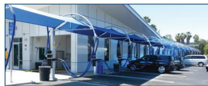
Vacuum booms with dual drops with canopies
