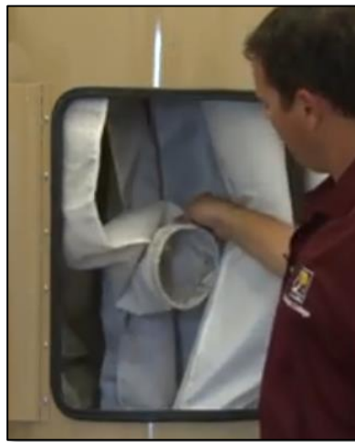
Example of an un-seated filter bag.
