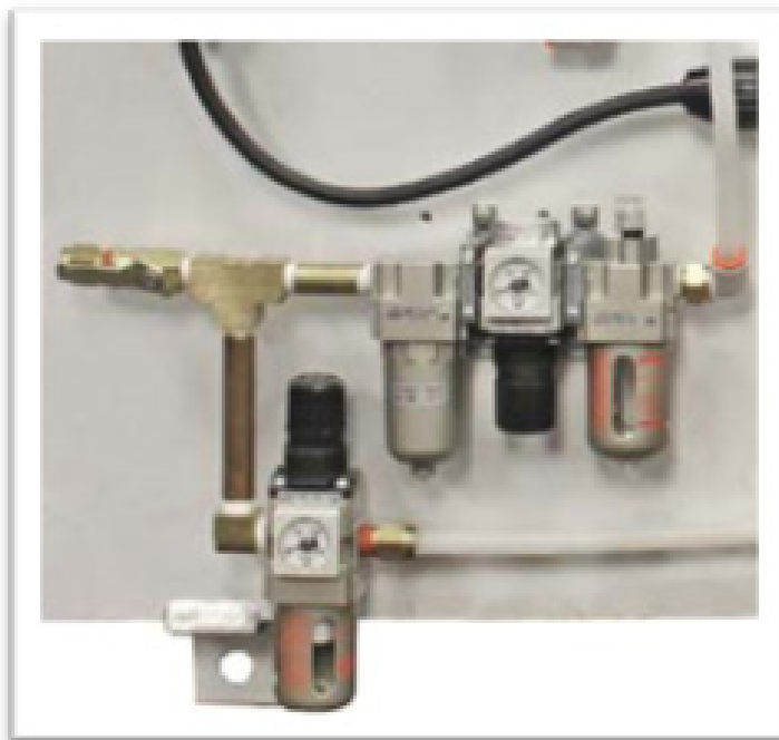
Figure 17. TSA Panel FRL Assembly Parts List
