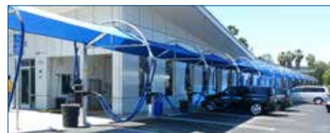
Vacuum booms with dual drops with canopies
