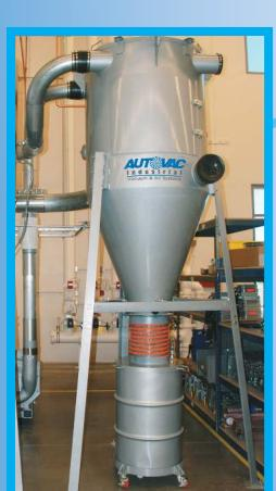
Next you'll need to separate the dirt and debris from the airflow before it returns to your vacuum producer. In standard central systems this is accomplished with a filter separator immediately before the air enters your turbine. Larger systems call for the addition of primary separators near the vacuum users. In each separator, waste is deposited into convenient dirt containers for easy disposal.
