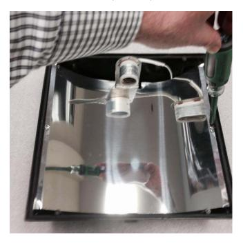
Disconnect wires from inside of lighting fixture and pull wires from junction box on vertical stanchion.
